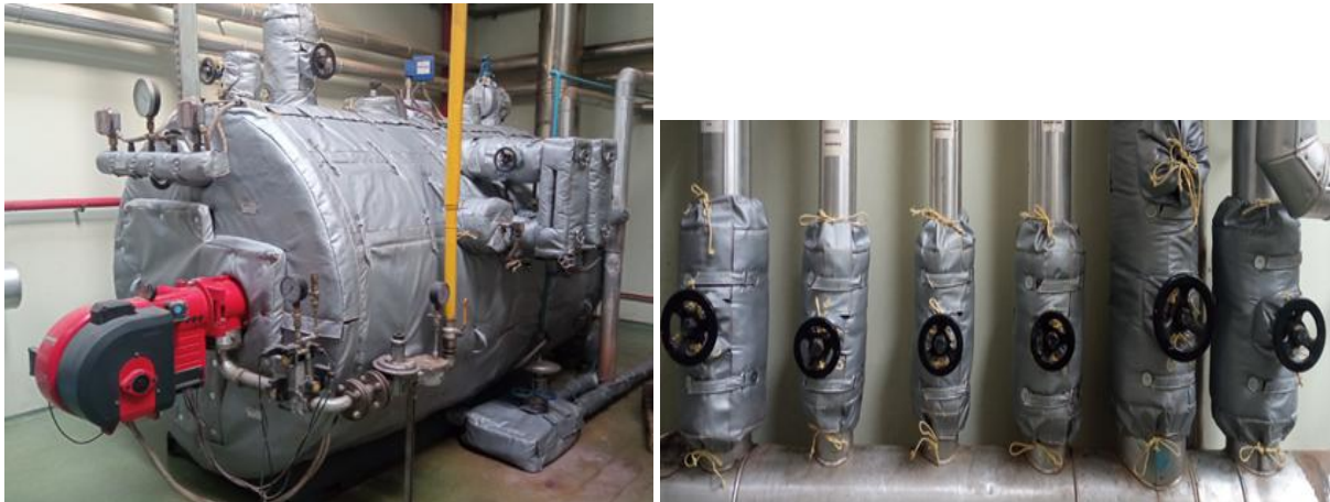
Fig. 13 – Energy efficiency through insulation mats at MartinBauer Germany
